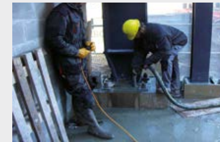
Filling steel columns
