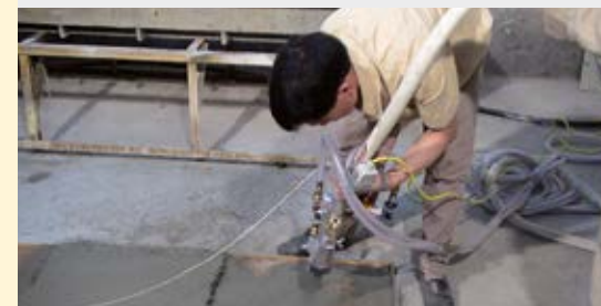
Making fibre-reinforced concrete slabs
