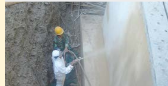
Coating concrete foundations
